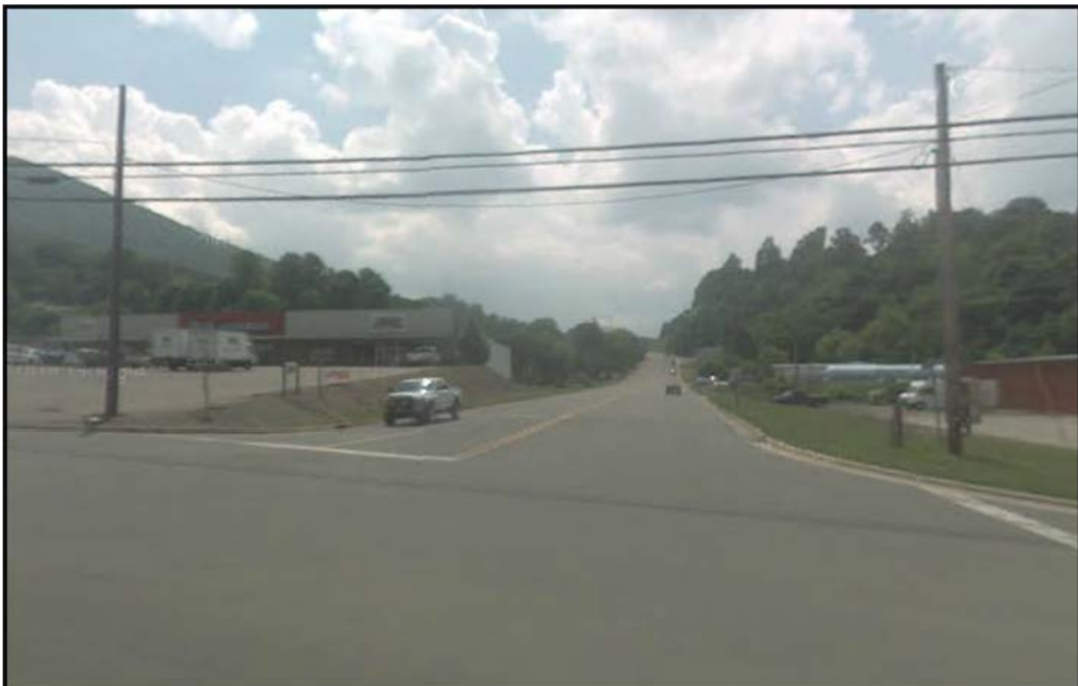
Google Maps (June 2009) – Looking South on SR 1149/Mount Jefferson Rd Approach
